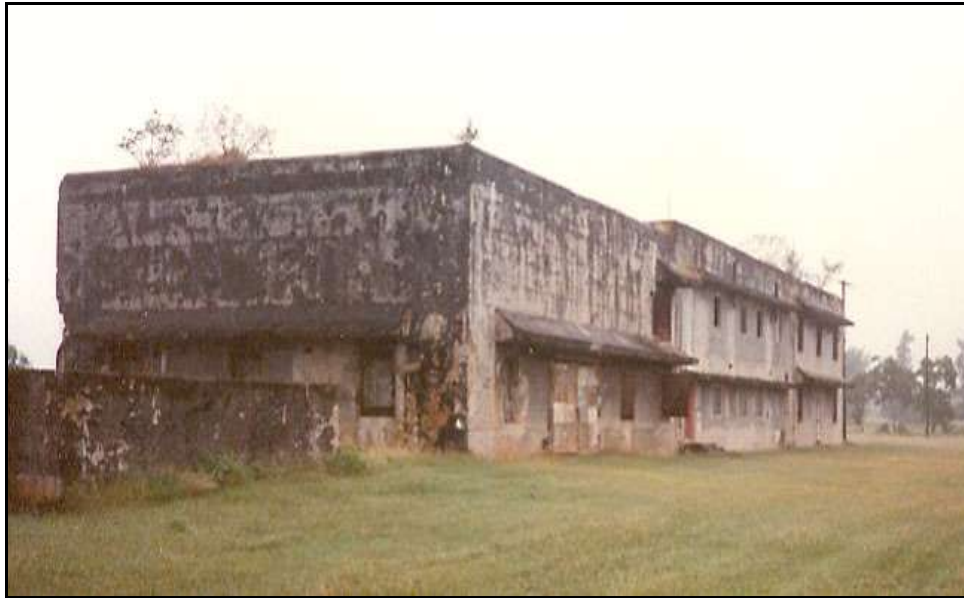
Figure 13.1-16. The WWII Era Japanese Radio Communications Center
