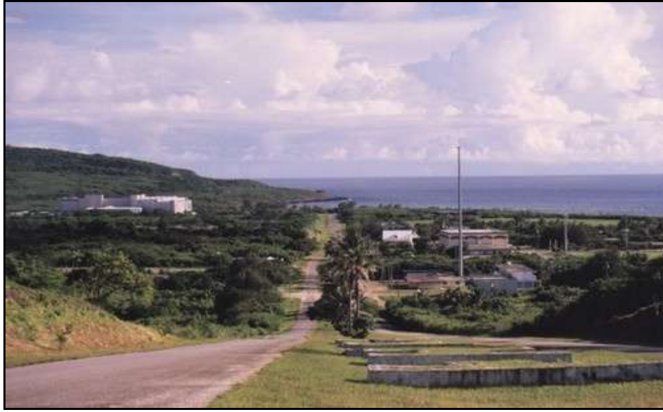
Figure 13.1-17. A View of San Jose Village from 8th Avenue Tinian Dynasty Hotel can be Seen on the Left Side of the Photo with the Tinian Channel Beyond
