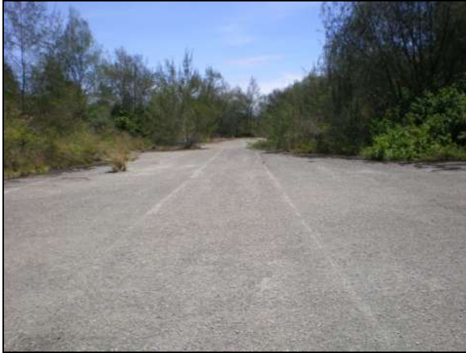
Figure 13.1-4. View of Degraded Airfield and Overgrown Vegetation Source: EDAW 2009.
